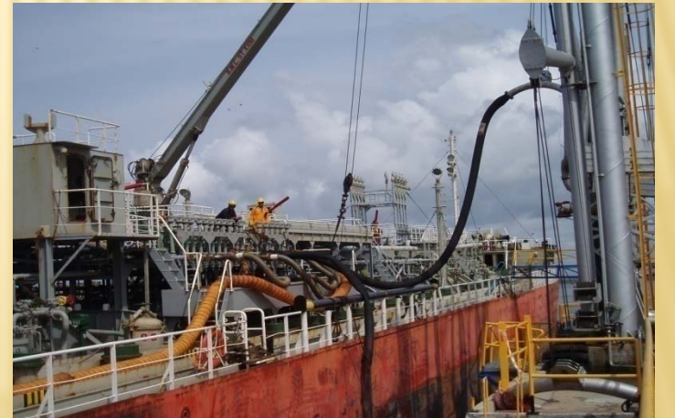
Quai principal Appontement
