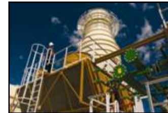
Gas 1 at Ankerlig (and Gourikwa) in the Western Cape
