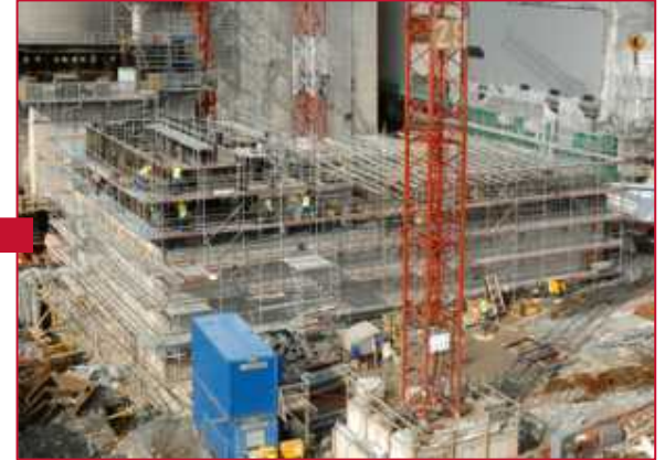
Diesel Building (UBP)
