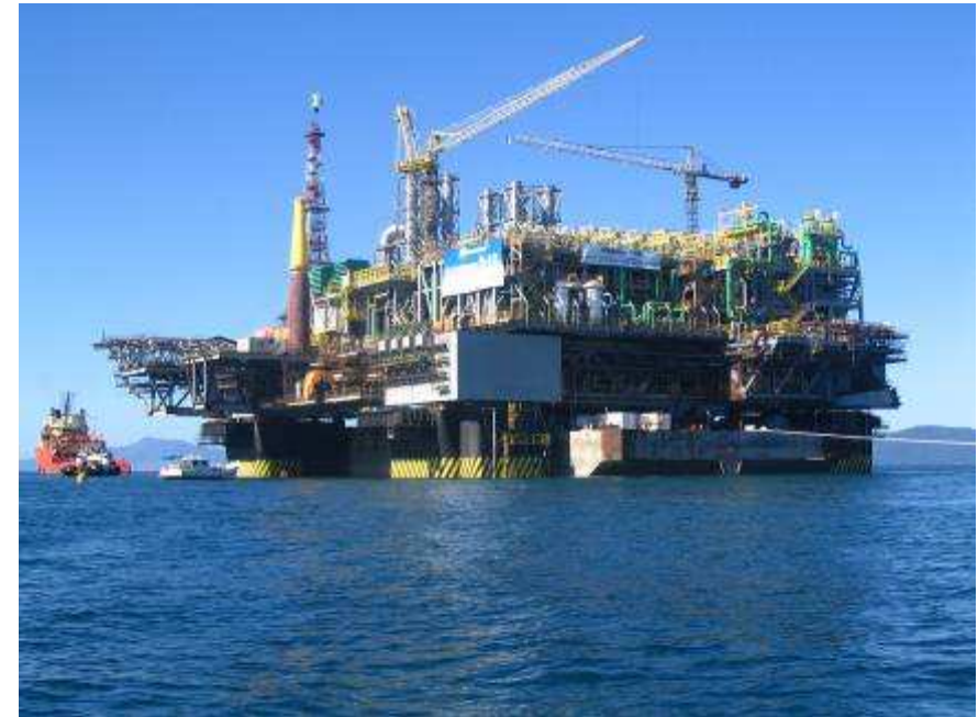
P-52 semi-submersible platform mating operation
